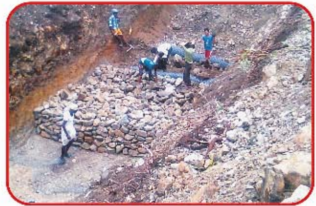
Gabion Bandhara Using Local Material
